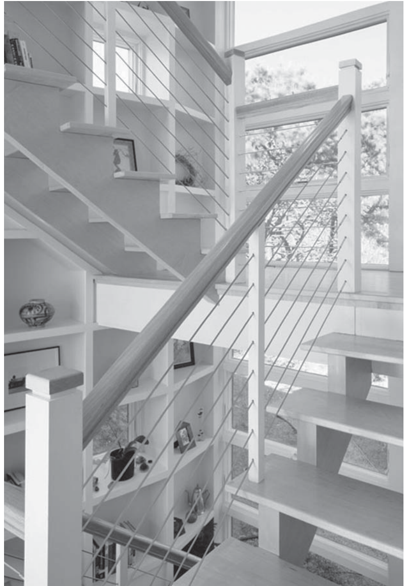
All Feeney cables and fittings are grade-316 (Marine Grade) Stainless Steel
