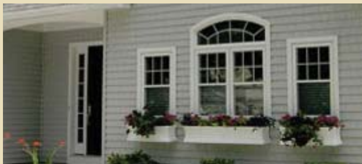
Segmental shape mullied to a pair of double hungs
